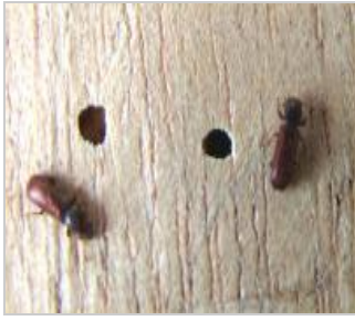
Powder post beetle and emergence holes
