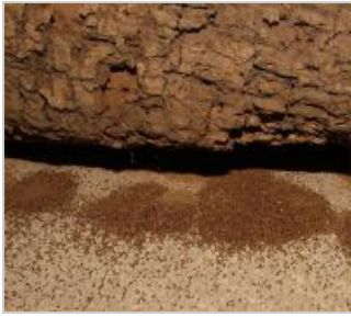
Death watch beetle damage and frass
